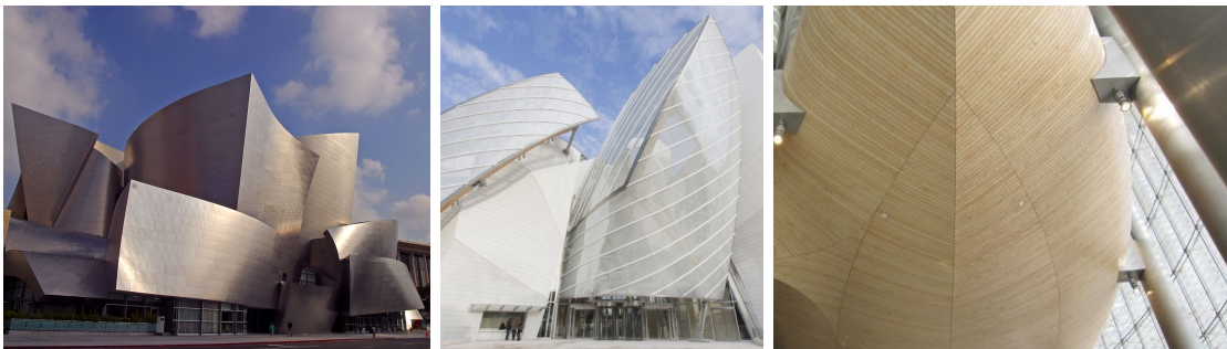
FIGURE 1. Freeform skins composed of developables. Left: The Disney Concert Hall consists of large near-developable pieces. Center: The Fondation Louis Vuitton, Paris, is composed of strip sequences, each strip being made from cylindrical glass panels and approximating a continuous developable. Right: The interior of the Burj Khalifa, Dubai, exhibits a paneling by “geodesic” developable elements, using the terminology of (Pottmann et al., 2008) and (Wallner et al., 2010). All three designs are by F. Gehry.
