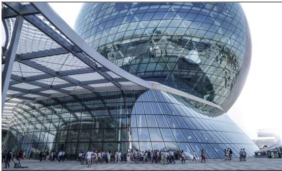
Figure 6: Side detail of Nur Alem , the main pavilion of the Astana EXPO 2017 Exhibition in Astana, Kazakhstan. Mostly cylindrical panels were used to rationalize the curved transparent freeform façade (different from the sphere).
