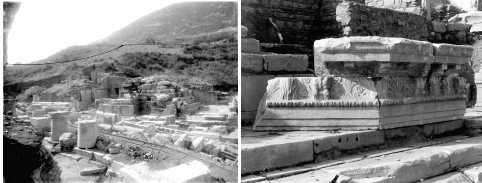
Fig. 3. Photos from the year 1905 showing components of the Octagon. The photo at right shows manually reassembled parts. (Photos are courtesy of the Austrian Archaeological Institute).
