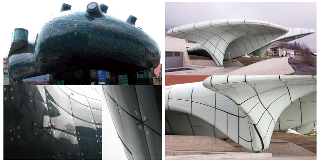
Figure 2: Projects involving double-curved panels where a separate mold has been built for each panel. These examples illustrate the importance of the curve network and the challenges in producing architectural freeform structures. (Left: Peter Cook and Colin Fournier, Kunsthau, Graz. Right: Zaha Hadid Architects, Hungerbergbahn, Innsbruck.)
