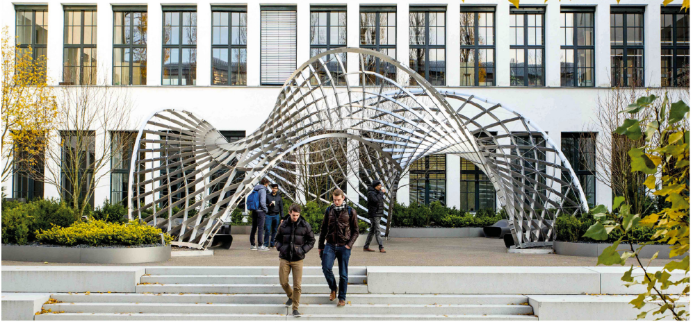
Figure 16: The Asymptotic Gridshell was completed in October 2017. The structure is 5 m high and spans 9 \times 12 m. It is built entirely from 1.5 mm-thick and 100 mm-wide steel lamellas. (Image: Felix Noe)
