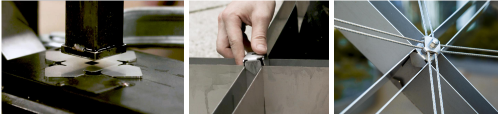
Figure 12: The typical grid joint is assembled with two parallel lamellas in each direction. Two standardized star-shaped washers fix the 90 degree intersection angle and create a central axis for the carriage bolt. The steel cables are also constructed in pairs and are fixed by a cross-shaped clamp. (Images: Felix Noe)
