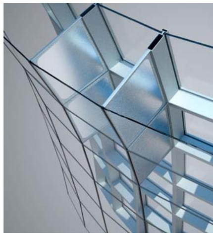
Multilayer structures are spatial patterns around a surface-like pattern. This image (courtesy Benjamin Schneider) shows a structure which is based on a conical mesh and formed by planar quads only.
