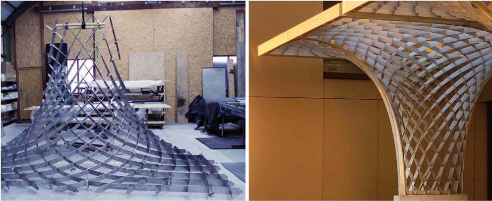
*Figure 17: Asymptotic Canopy for the Intergroup Hotel in Ingolstadt. The grid is designed with a transition from  $90$  to approximately  $60$  node angles, thus allowing for a bespoke shape and a directed load-path. Each segment prefabricated hanging upside down, to form the design geometry.*
