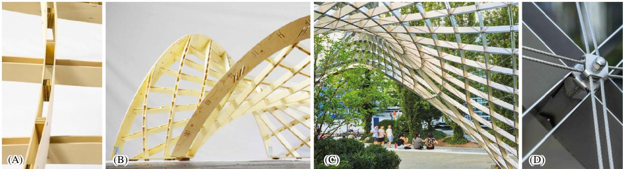
Figure 2: Gridshells using asymptotic networks. (A,B) The first asymptotic timber prototype was developed at the TUM in 2016, using double lamellas of laminated poplar and square timber studs. (C,D) In 2017, the Inside/Out Pavilion was built out of stainless steel lamellas, with repetitive 90-degree joints, and was braced with diagonal pre-stressed cables.
