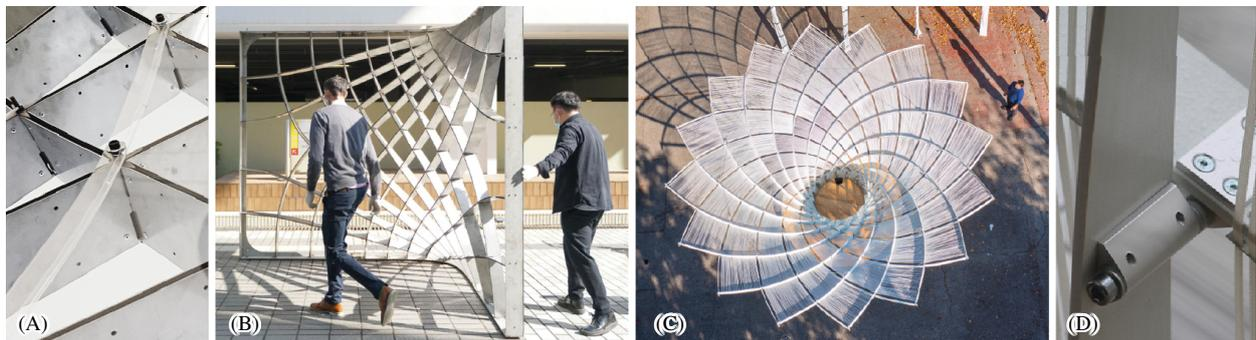
Figure 3: Asymptotic networks as façade and transformable structure. (A,B) The asymptotic building envelope prototype was built in 2020, to investigate the application as facade substructure. (C,D): The kinetic umbrella is a transformable structure using GRP lamellas and was completed in 2021.
