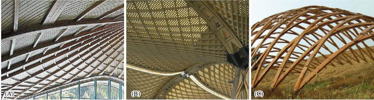
Figure 1: Timber Gridshells using geodesic planks. (A) The ribbed Gridshell in Bad Dürrenheim was built with a primary grid along the principal curvature lines and a diagonal cover of geodesic planks. (B) The Expo Hannover Gridshell (by Natterer & Herzog) combines laminated geodesic ribs with a diagonal geodesic substructure. (C) The deployable geodesic Almond Gridshell (by Soriano) was designed to allow a flat assembly and kinetic erection process.
